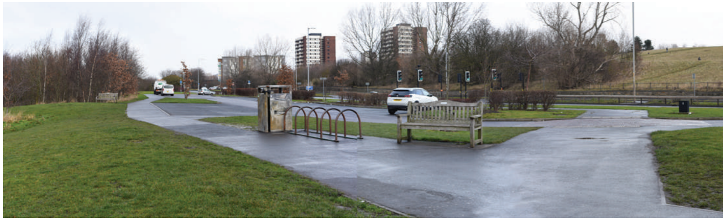
7 Entrance to car park on Durham Road (facing North). Street clutter dominates, with little design to car park edges considered.
